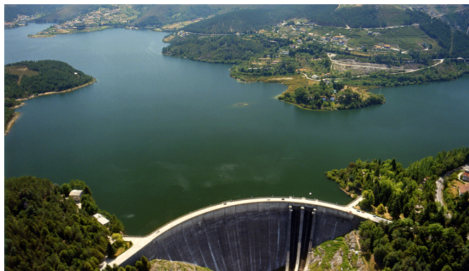
Figure 1.1: Aerial view of the Frades II power plant upper reservoir and dam.
