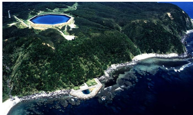
Figure 1.3: Aerial view of the Okinawa Yanbaru power station.
