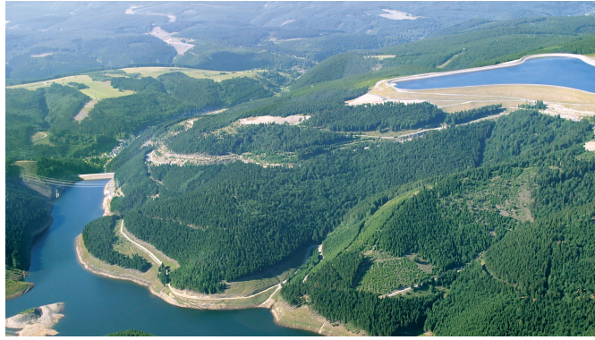
Figure 1.4: Aerial view of the Goldisthal Pumped Storage Power Plant.
